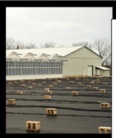
A compacted surface and an impermeable barrier will assist in collecting any nutrient rich water from your outdoor collection area.
